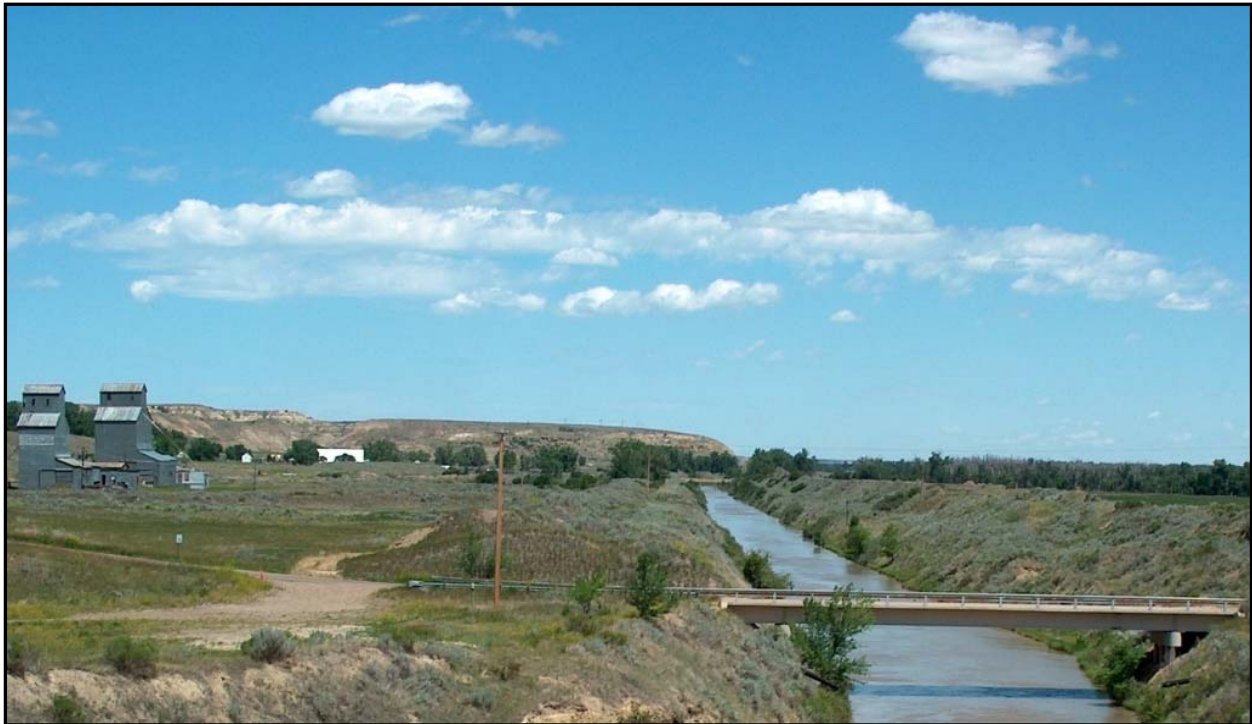
Overview of the Project area – looking north from the Intake headworks
