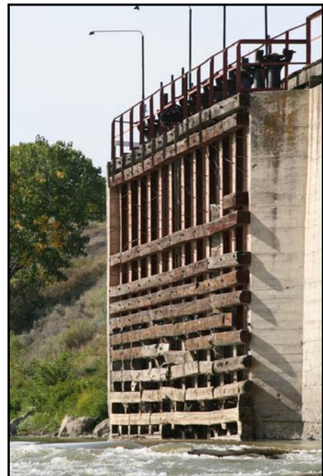
Existing unscreened main canal headworks
