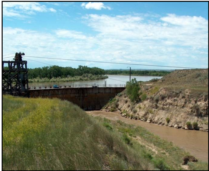
Lower Yellowstone main canal and headworks looking towards the Yellowstone River
