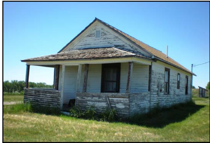
Headworks Gate Tender's Residence
