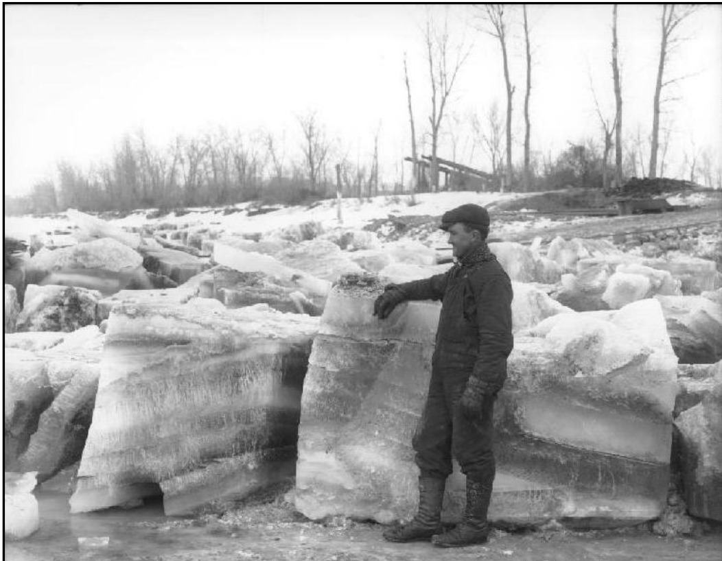
Ice blocks removed from Yellowstone River during construction of Lower Yellowstone Project
