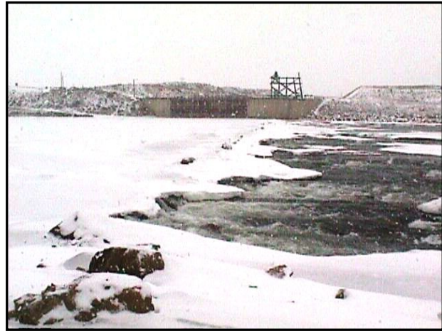
Winter at Intake Diversion Dam
